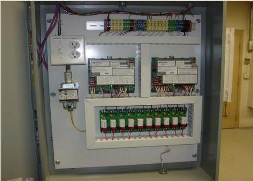
A receiving unit at the Fort Collins plant gets a signal from the utility about upcoming peak times (above) and the signal is fed to a programmable logic controller (below) to automatically shed non-essential loads.
