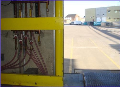
*Hot glycol lines need to be cooled. Snow on the northern loading docks needs to be melted. Solution: running the glycol lines under the loading docks fixes both problems with minimal energy use.*
