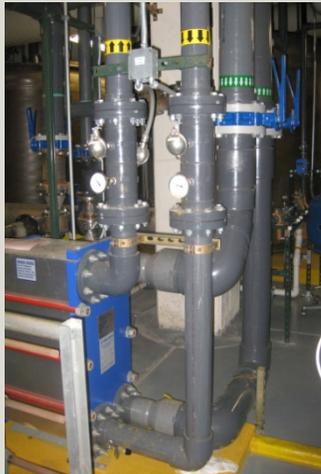
*Instead of using natural gas to heat incoming city water, Avago redirects excess heat from the chiller condenser to accomplish the same purpose.*
